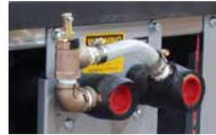
Typical optional automatic low flow bypass valve.
